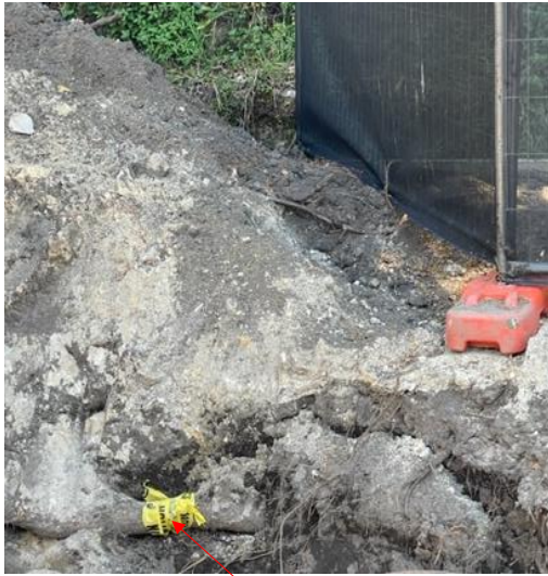
Photo C: Tree 7 and one 90mm root requiring pruning outside of the TPZ area (fencing in photo).
